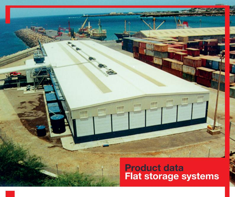
A flat storage offers low capital cost and quick installation compared to conventional silos. Each system is tailormade to fit an existing or new storage building. The loading and unloading systems can be manual, semi-automatic or fully automatic.
