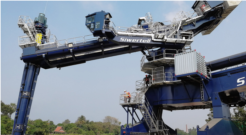
SHIP UNLOADER - THAILAND
