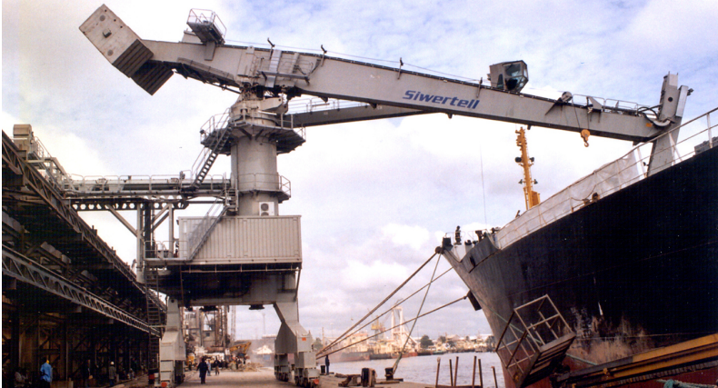
SHIP UNLOADER - NIGERIA
