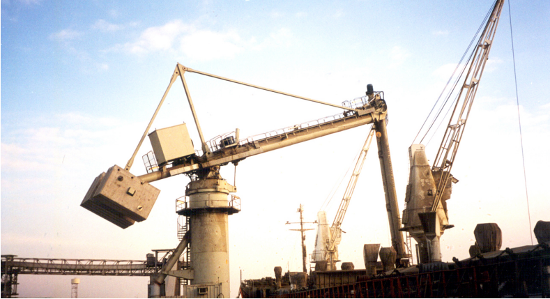
SIWERTELL SHIP UNLOADER - EGYPT
