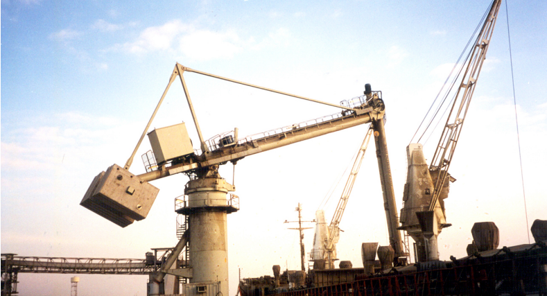
SHIP UNLOADER - EGYPT
