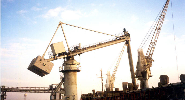
SIWERTELL SHIP UNLOADER - EGYPT
