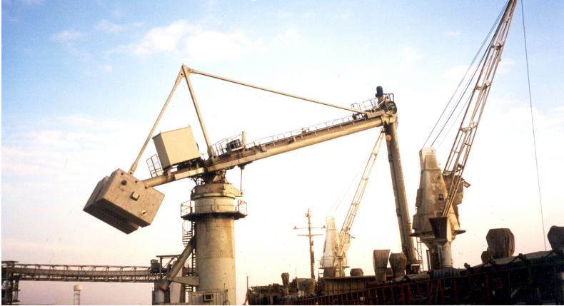
SHIP UNLOADER - EGYPT
