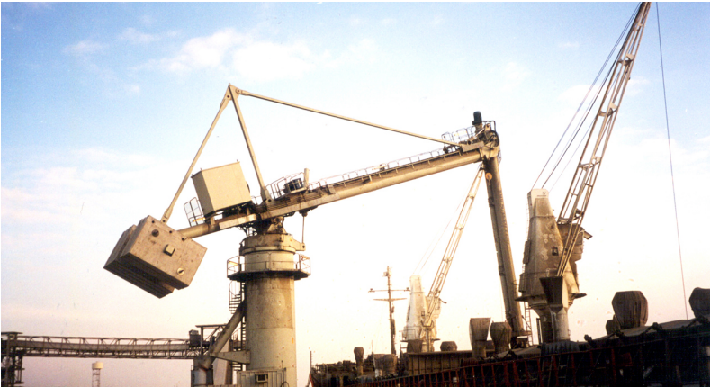
SHIP UNLOADER - EGYPT
