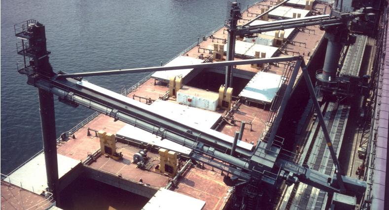
SHIP UNLOADER - NETHERLANDS
