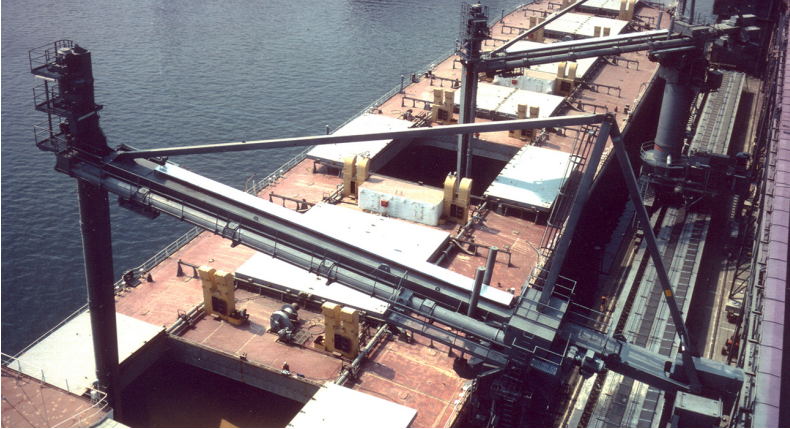
SHIP UNLOADER - NETHERLANDS
