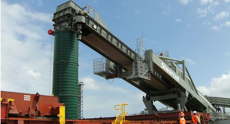
SIWERTELL TERMINAL - AUSTRALIA
