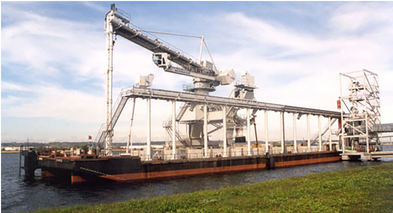
SIWERTELL TERMINAL - FRANCE
