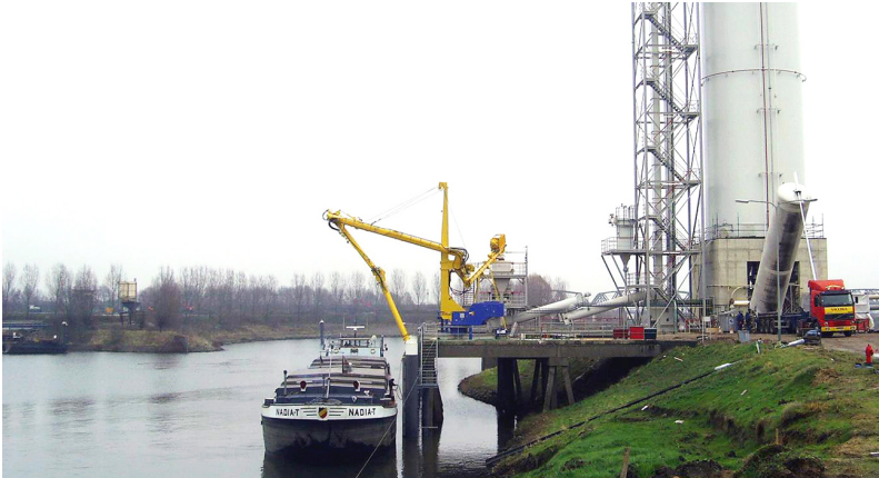
MOBILE UNLOADER - NETHERLANDS
